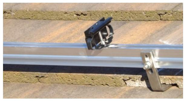
Finally, the first solar panel can be fitted into position. Four clamps are used to hold a solar panel into position. However, each clamp can hold two solar panels down when the panels are next to each other.
