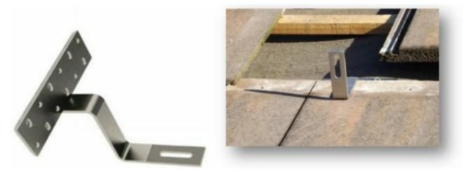
To install solar panels onto an existing tiled roof, individual tiles are slid out and a roof hook is fitted beneath the tile, mounting directly onto the underlying roof truss. Once mounted, the original tile can be slid back into position. Depending on the type of tile and the roof hook design, it may be necessary to chisel out part of the underside of the tile in order to achieve a good fit.
