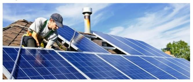
Solar panels or, more accurately, *photovoltaic* solar panels, generate electricity from the sun. The more powerful the sun's energy, the more power you get, although solar panels continue to generate small amounts of electricity in the shade. Most solar panels are made up of individual solar cells, connected together. A typical solar cell will only produce around half a volt, so by connecting them together in series inside the panel, a more useful voltage is achieved.
